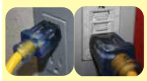
Plug into grounded outlets. DO NOT use if ground plug is broken.
